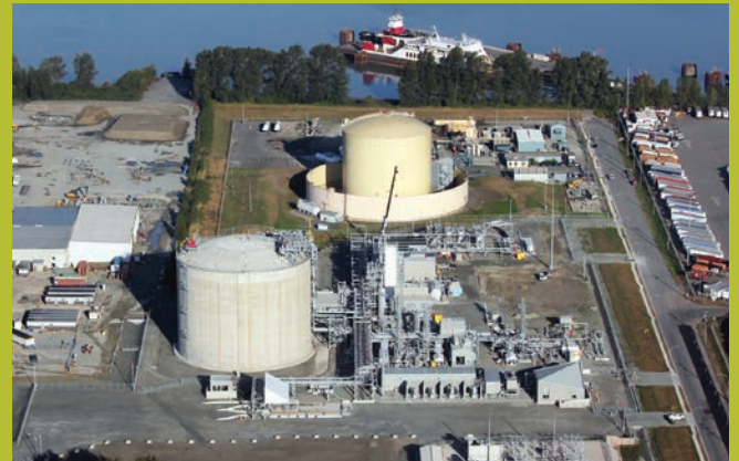
FortisBC's LNG facility in Delta, BC has been operating since 1971 and in order to meet the growing demand for LNG it recently underwent a $400-million expansion.
