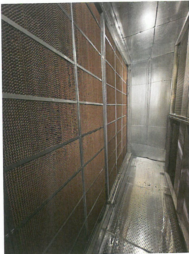
An Evaporative Pad Humidifier installed in AHU (upstream). Armstrong International
