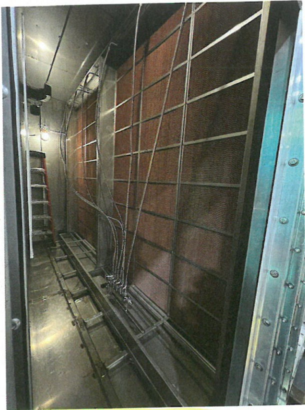
An Evaporative Pad Humidifier installed in AHU (downstream). Armstrong International
