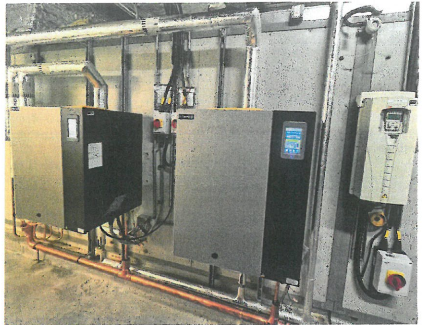
Compatible with all water types, DriSteem's RTS humidifier continuously learns as it runs and automatically adapts to optimize steam output and overall performance. DriSteem
