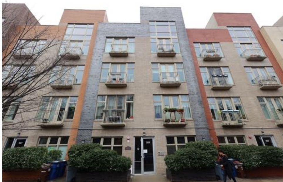
A series of attached five-story single-exit buildings built in Brooklyn, NY, in the 2010s, per NYC BC 1006.3.2.7 (photo by Andressa Randis, used with permission)
