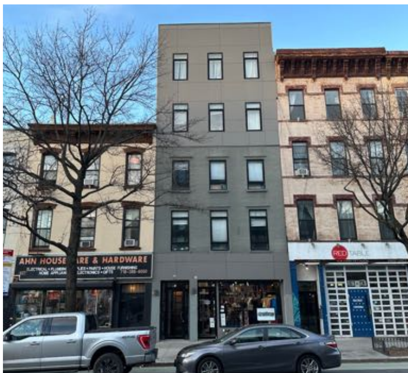
Proponent's condo building, featuring seven dwelling units over one store, outfitted with NFPA 13R sprinklers and served by a single exit, per New York City Building Code 1006.3.2.7 (photo by author)
